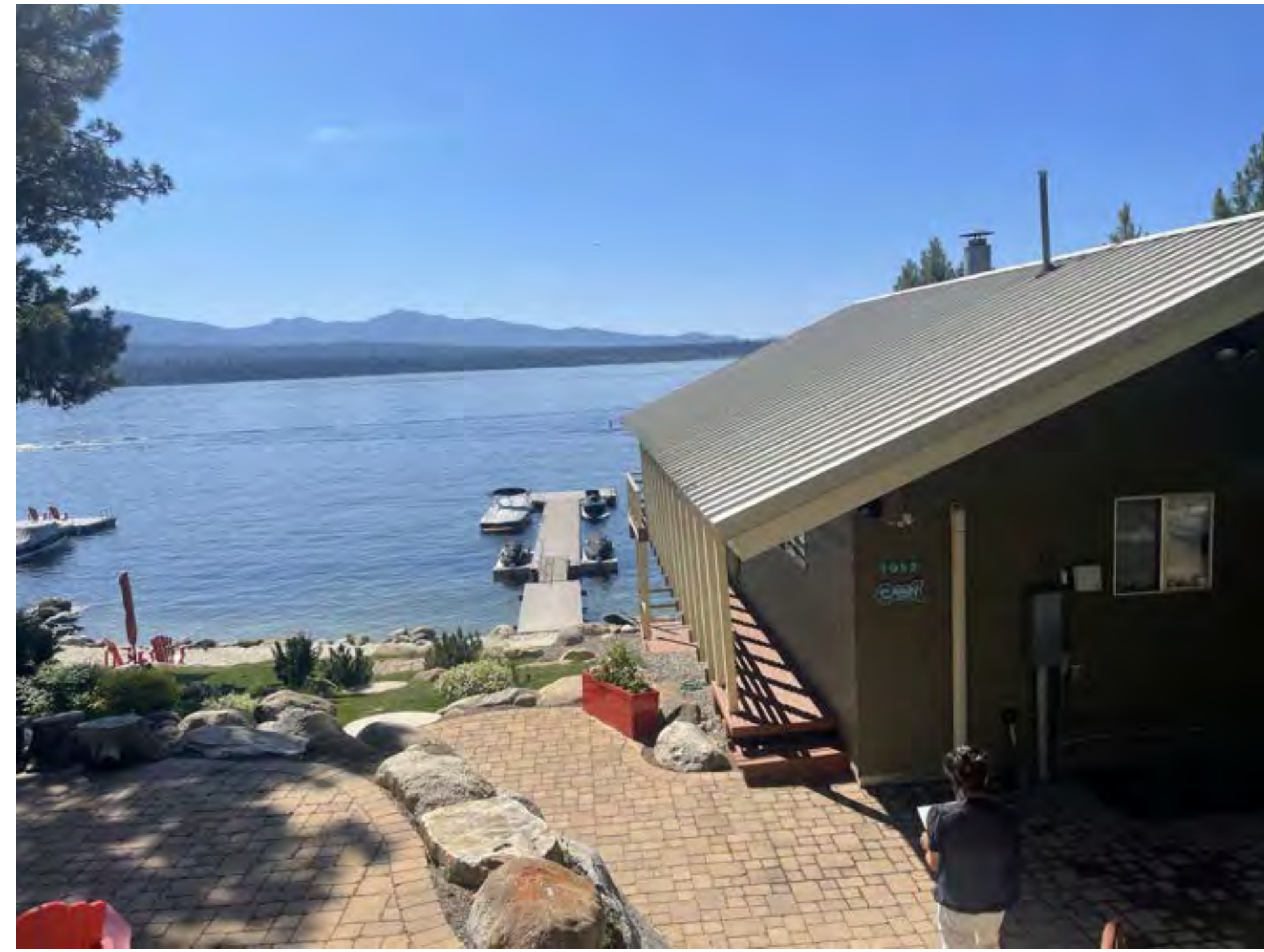
2 EXISTING NON-CONFORMING HOME
