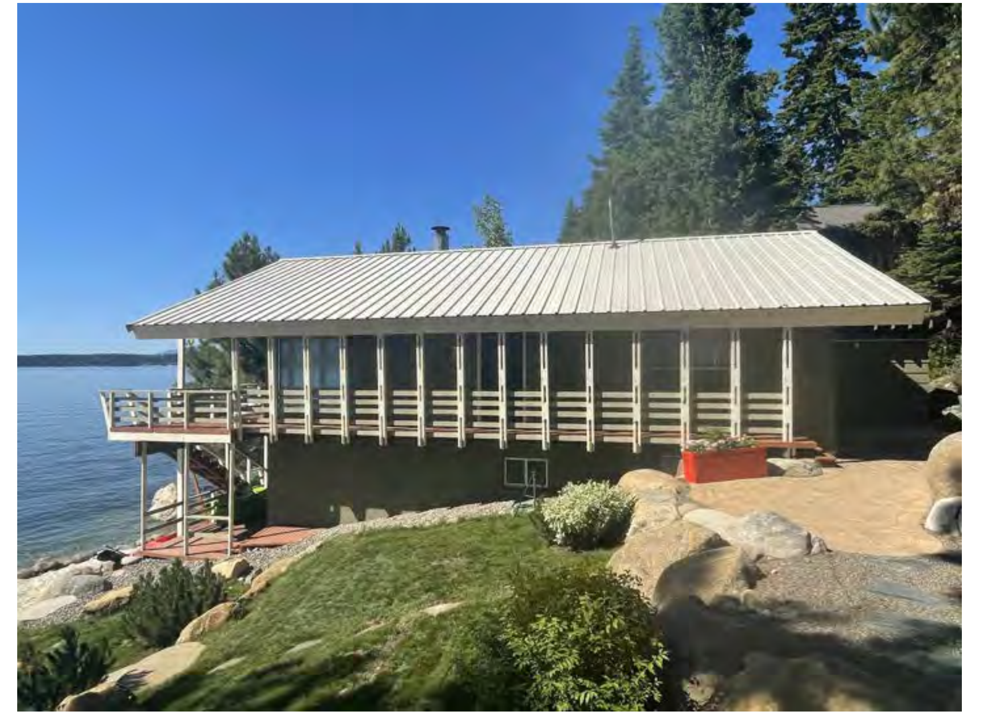
3 EXISTING NON-CONFORMING HOME
