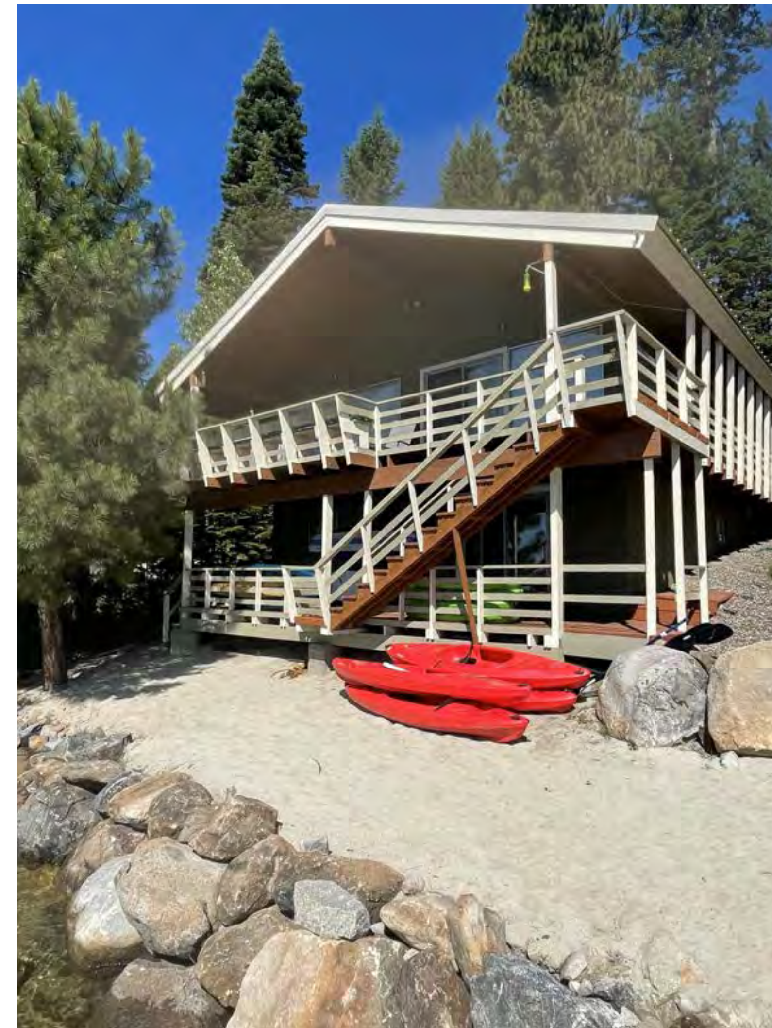
5 EXISTING NON-CONFORMING HOME
